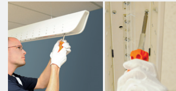
2. Unscrew the entire LED assembly from the housing.
