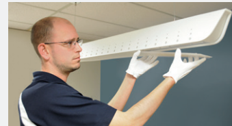
1. Lift and shift or remove the lens.
