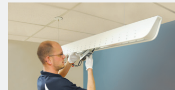
6. Remove the LED driver and replace.
