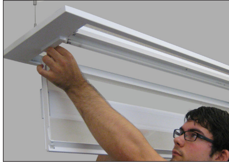
While supporting the doorframe from below, detach the retention strap from the housing (at fixture end) by sliding sideways towards the center of the fixture and pulling out of the slot. Repeat at opposite end of fixture.
