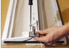
Slide bracket into end of fixture. Attach bracket to fixture using supplied washers and screws.
