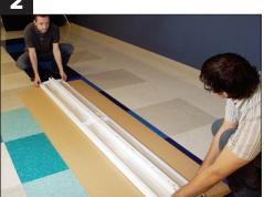
Arrange boxed fixtures on floor in specified mounting locations; remove fixtures from boxes; remove plastic from fixtures.
