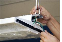
POWER LOCATIONS: Feed power cord through bushing (shown above). Complete electrical connections using wire nuts (supplied by others).
