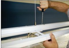
Secure in-run bracket from above using supplied screws (requires Phillips screwdriver). LEVEL FIXTURE: Ensure fixture is level end-to-end. Support fixture from below and use supplied aircraft cable release tool to make fine height adjustments. Trim aircraft cable below adjuster as required.
