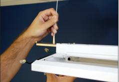
With two people, raise first fixture to ceiling. At each end of fixture, insert aircraft cable through aircraft cable adjuster (located on mount bracket). The adjuster will automatically grip and hold the cable.
