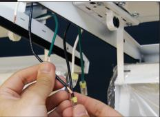
Complete in-run electrical connections. NON-POWER LOCATIONS (shown above): Use supplied guickwire connectors. Tuck wires into wire cavity. POWER LOCATIONS (shown in STEP 6): Feed power cord through bushing in bracket. Use wire nuts (supplied by others to complete connections. Tuck wires into wire cavity.
